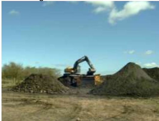
Screening soil for ex situ amendment
